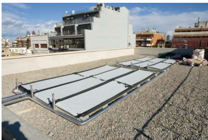
24m 2 of flat solar thermal collectors
